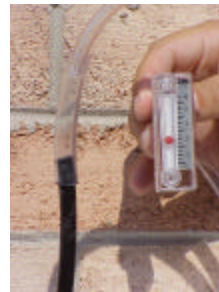
Cut Excess AFCI™ & push 2" - 3" Inside Tube
