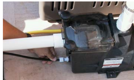
Strainer Basket Installation
