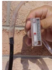
Cut Excess AFCI™ & push 2" - 3" Inside Tube
