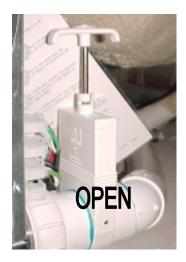
Make sure the filter cartridge (basket and weir, if so equipped) is in place. Fill the spa using a garden hose until the water is halfway up the "throat" of the skimmer, otherwise it will suck air, which will cause the pump motor to "run dry" and burn up. This repair would not be covered under warranty. You should check the water level of your spa each day as there is normal evaporation each day, and more often when spa is used frequently.
