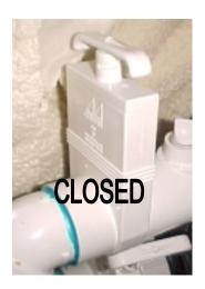
All gate valves must be OPEN. There are two twist and turn locking gate valves located under the skirt on each side of the Equipment Pack.
