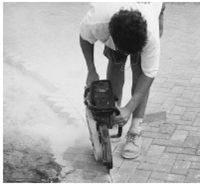
Figure 8. Saw cutting pavers.
