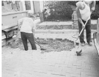
Figure 2. Removal of concrete pavers for a gas line repair in Dayton, Ohio.
