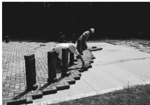
Figure 7. Placing the concrete pavers.
