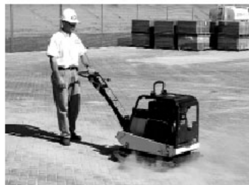
Figure 12. Final compaction should consolidate the sand in the joints of the concrete pavers.
