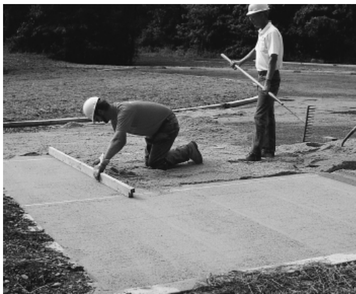
Figure 6. Screeding the bedding sand.
