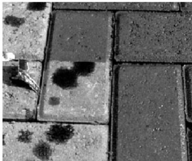
Figure 9. Sealers resist stains which makes them ideal for high use areas where they might occur.
