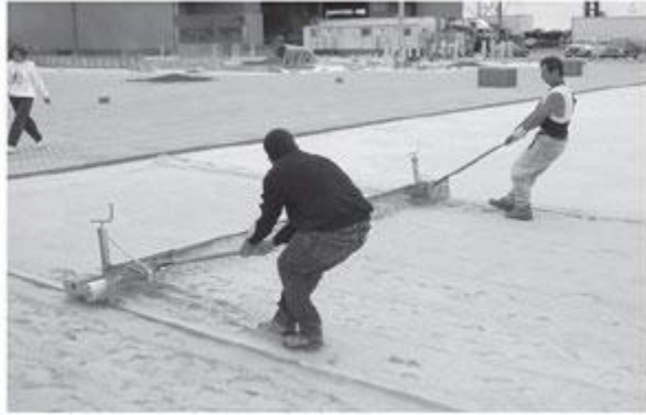
Figure 4. A two-man hand pulled screed
