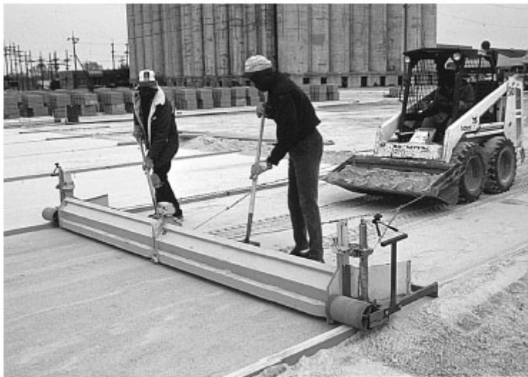
Figure 17. Powered screed bucket accelerates spreading of bedding sand. The width of the bucket can be adjusted.
