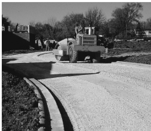
Figure 4. Base compaction with a vibratory roller.
