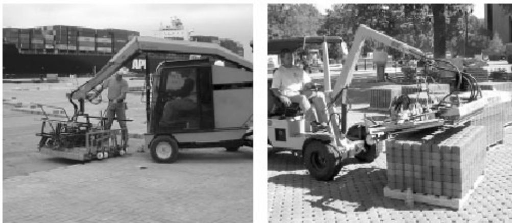
Figure 1. Mechanical installation of interlocking concrete pavements (left) and permeable units (right) is seeing increased use in industrial, port, and commercial paving projects to increase efficiency and safety.
