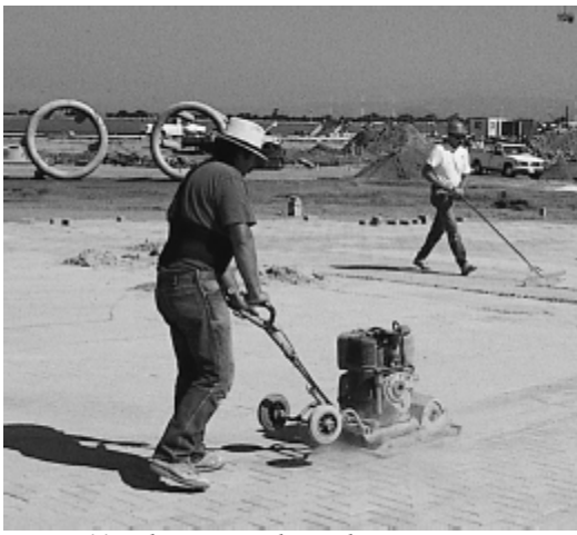
Figure 11. Vibrating sand into the joints.
