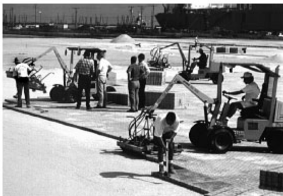
Figure 9. Mechanical installation equipment places concrete pavers rapidly.
