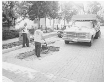
Figure 3. Compaction of the base.
