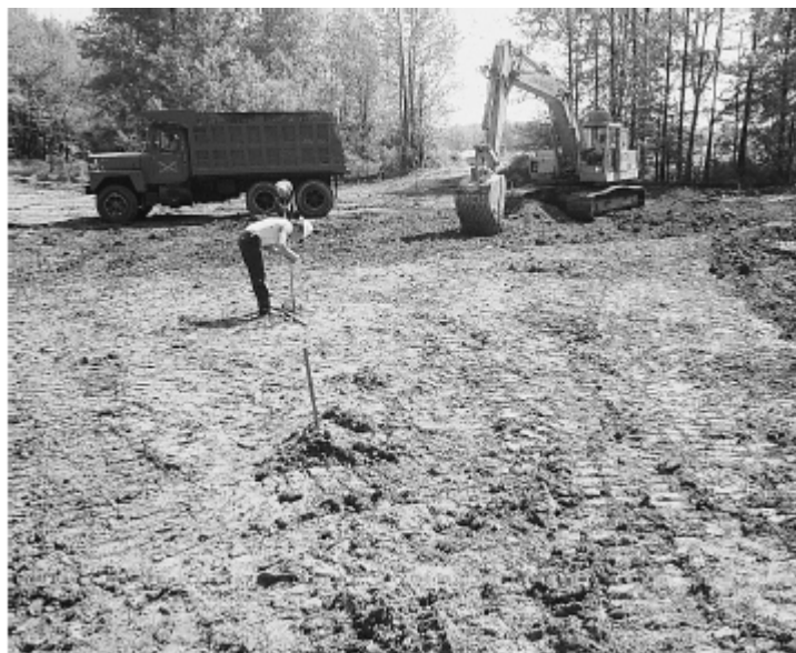
Figure 1. Excavation of the soil subgrade.
