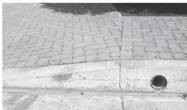
Figure 3. Ramp pavers changing angle.
