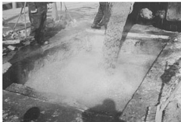
Figure 11. Low density concrete fill (unshrinkable fill) poured into a utility trench from a ready-mix concrete truck.
