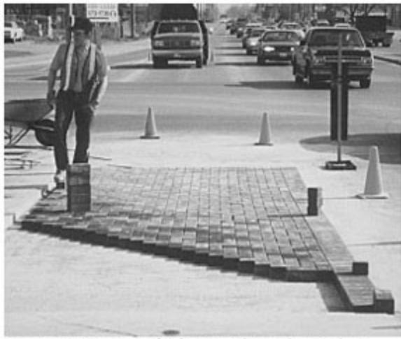
Figure 12. Pavers are laid in a 90 degree herringbone pattern between the border courses.
