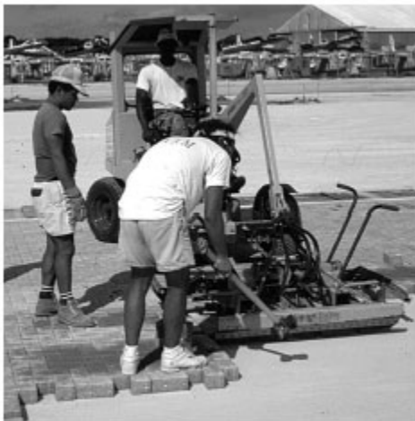
Figure 5. Motorized equipment with a hydraulic clamp.
