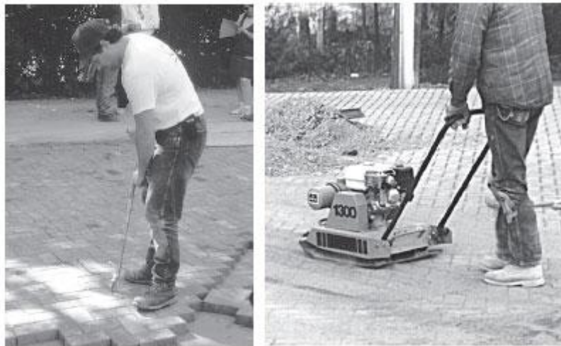
Figure 13 (Left). Adjusting joint spacing and alignment. Figure 14 (Right). Second and final compaction of the pavers. The first compaction occurs after the pavers are placed (no sand in the joints). The second compaction works the sand on pavers into the joints. This process causes the pavers to interlock.
