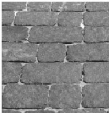
Figure 4. Liquid joint sand stabilizers can deepen the surface color slightly and they provide some surface sealing as well. Tumbled pavers shown here have wider joints than other shapes. These type of pavers can require stabilization of the joint sand.
