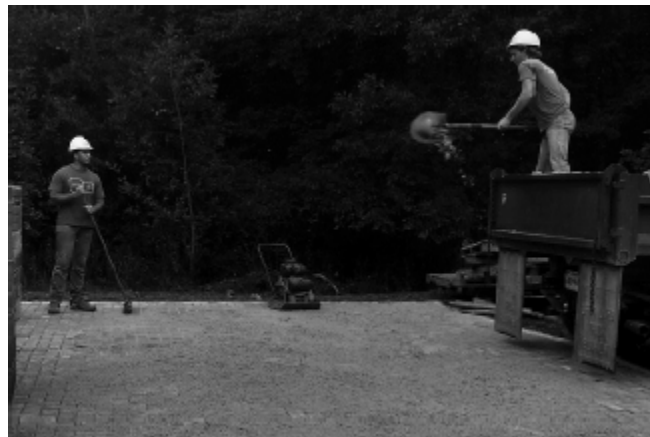
Figure 10. Spreading and sweeping joint sand.
