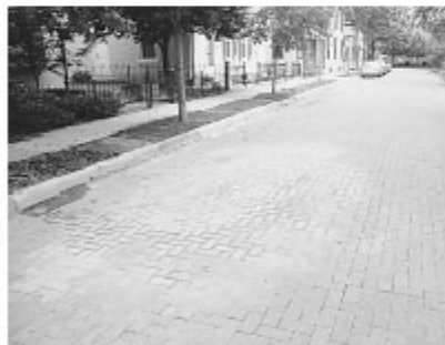
Figure 5. The final paver surface is continuous. There are no cuts or damage to the pavement.
