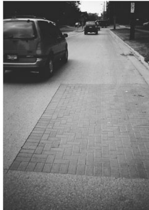
Figure 8. Utility cut repair in a residential area in London, Ontario.
