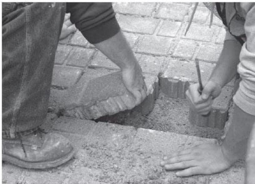
Figure 7. Pulling out a paver by the short end provides greater leverage and makes extraction easier.
