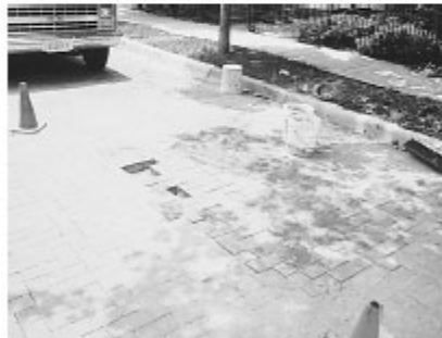
Figure 4. Reinstatement of the pavers, bedding and joint sand.
