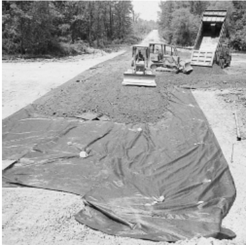
Figure 3. Application of the geotextile under aggregate base.
