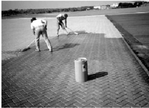
Figure 10. Urethane is applied with squeegees to stabilize joint sand between pavers on aircraft pavement.
