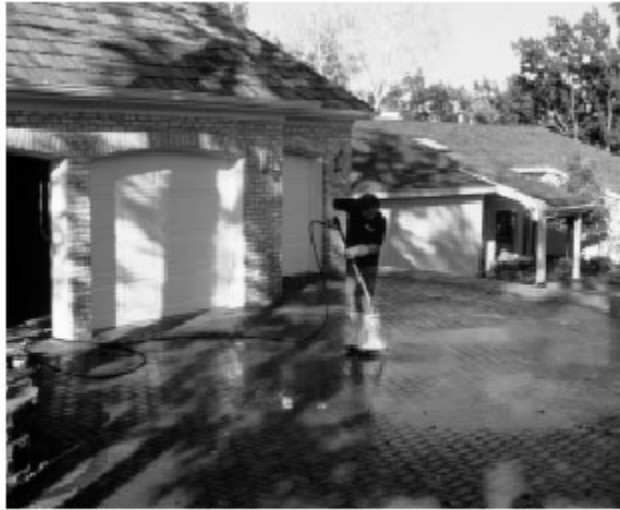
Figure 2. Pressurized cleaning equipment used by professional cleaning and sealing companies can bring out the best appearance from pavers.
