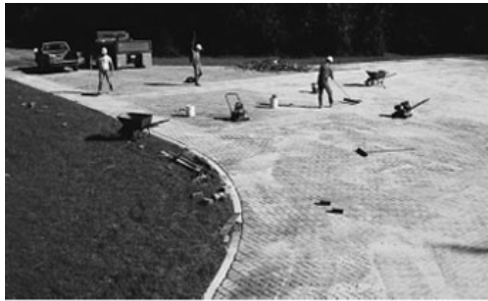
Figure 12. Excess sand swept from the finished surface will make the pavement ready for traffic.
