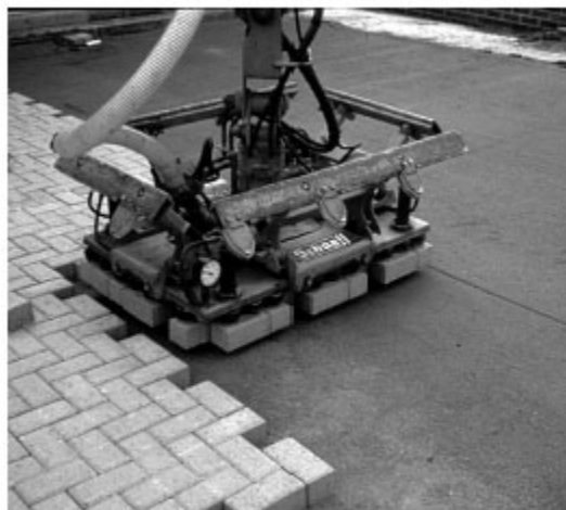
Figure 6. The vacuum head over the paver layer.
