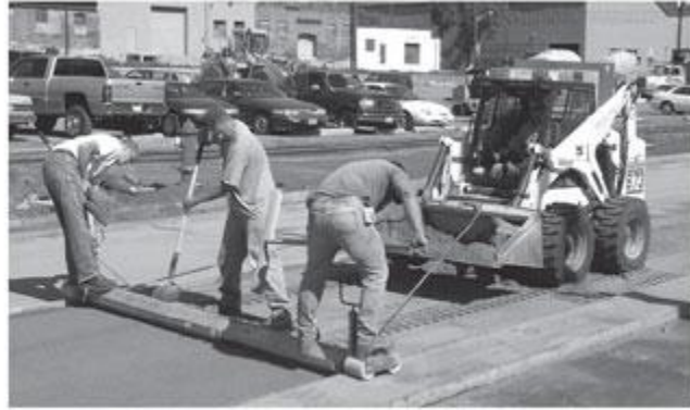
Figure 5. Mechanical screeding is the most efficient method of bedding sand installation
