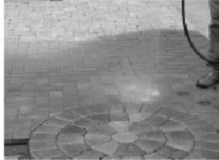
Figure 7. Dry-applied joint sand with a stabilizer is wetted in order to activate it and stiffen the sand. Once the joints dry, they are stabilized.
