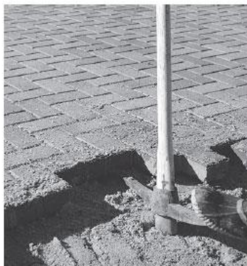
Figure 6. Prying out the remaining pavers
