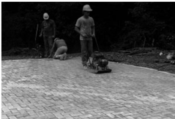
Figure 9. Compacting the pavers and bedding sand.
