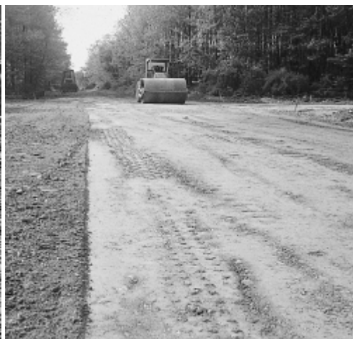
Figure 2. Compacting the soil subgrade.
