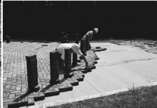
Figure 7. Placing the concrete pavers.
