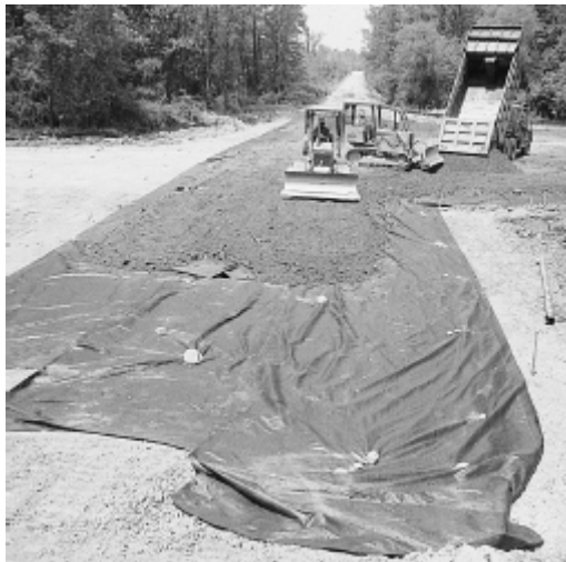
Figure 3. Application of the geotextile under aggregate base.
