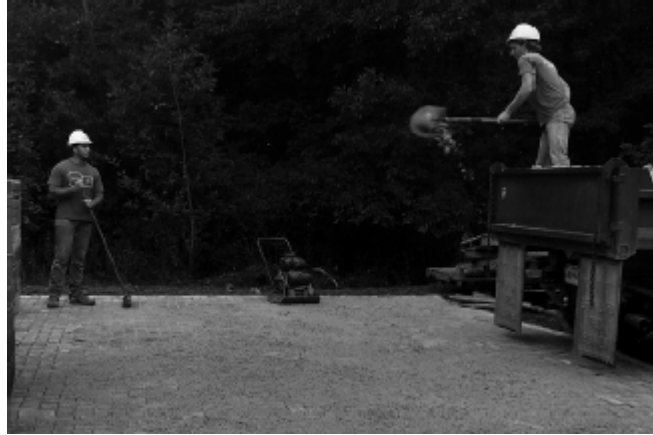
Figure 10. Spreading and sweeping joint sand.
