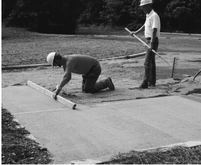
Figure 6. Screeding the bedding sand.
