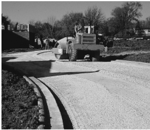
Figure 4. Base compaction with a vibratory roller.
