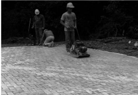
Figure 9. Compacting the pavers and bedding sand.
