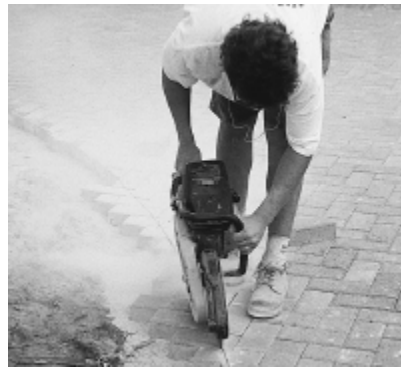
Figure 8. Saw cutting pavers.
