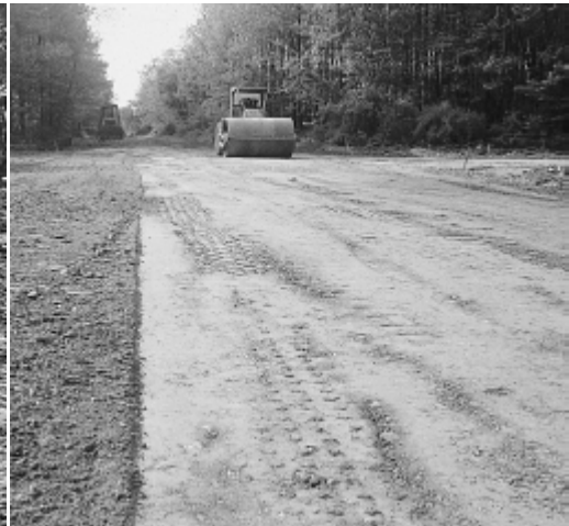
Figure 2. Compacting the soil subgrade.
