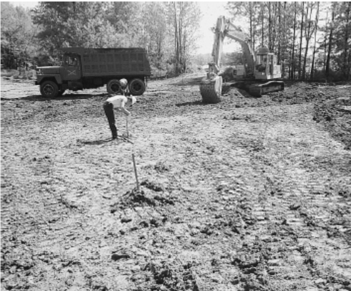
Figure 1. Excavation of the soil subgrade.
