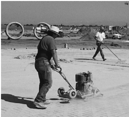
Figure 11. Vibrating sand into the joints.
