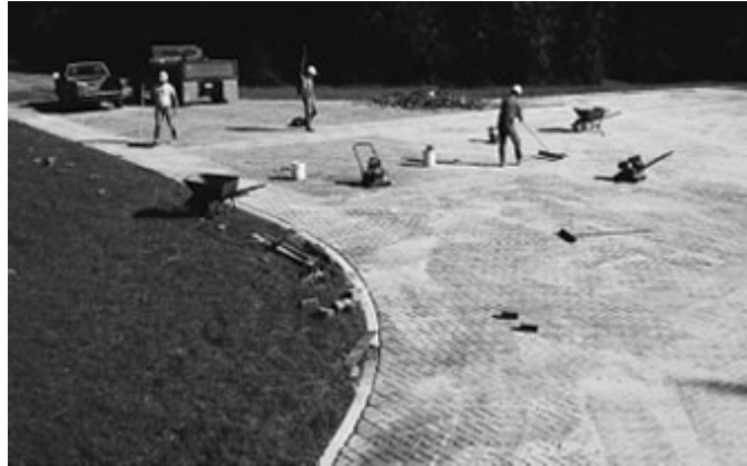
Figure 12. Excess sand swept from the finished surface will make the pavement ready for traffic.
