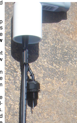
Water Sensor bent to jog away from cables and point downward. Zip-tie in final position
