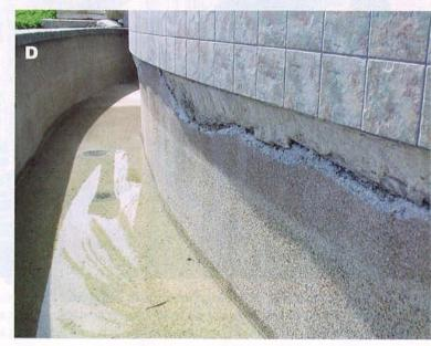
proper waterproofing should be enough to keep these exposed walls from failing.
