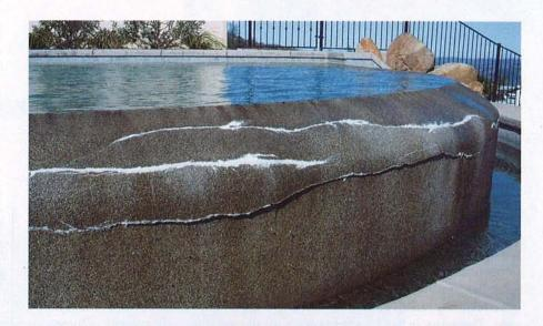
In the years since vanishing-edge pools gained incandescent popularity in the 1990s, we've seen more and more failures of the sorts depicted here, with extensive, disastrous cracking and delamination of surface materials. It took a while, but eventually patterns emerged that helped us determine why these freestanding weir walls were failing — and what needed to be done to prevent it.
