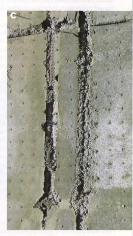
Workmanship plays a definite role in these problems with weir walls. Situations in which cages are inadequately secured and are able to move during shotcrete application are trouble (A), for example, as are instances in which no spacers are used to make certain rebar can be fully and completely encapsulated in concrete (B). The consequences in the latter case show up as soon as the forms are stripped (C) – and the situation only gets worse when water is introduced.
