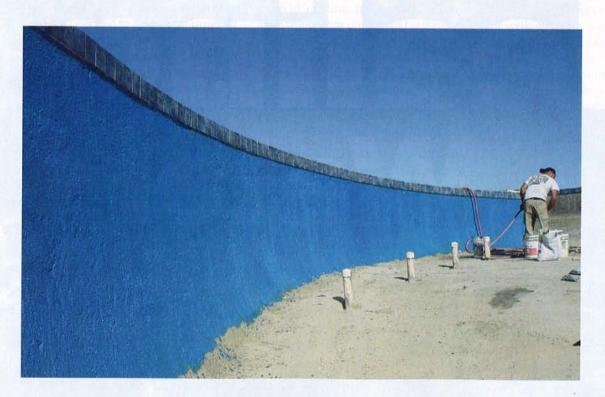
Waterproofing is a good idea on both sides of a vanishing-edge weir wall, simply because, when properly applied according to manufacturer instructions, these coatings minimize the transfer of water from the pool to the outside of the wall and thereby act as welcome layers of protection.
