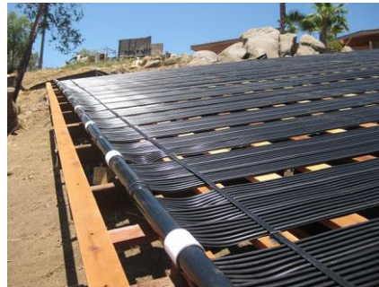
ALTERNATING MANIFOLDS - MALE TO MALE VIA PVC COUPLING FEMALE TO FEMALE VIA PIPE STUB
