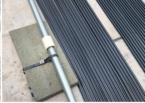
Strap under fin tubes first
