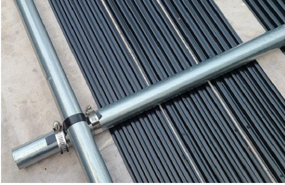
Cross rail over fin tubes last
