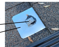
HOT SUN STRAP BRACKET 3"x6" AL ROOF FLASHING
