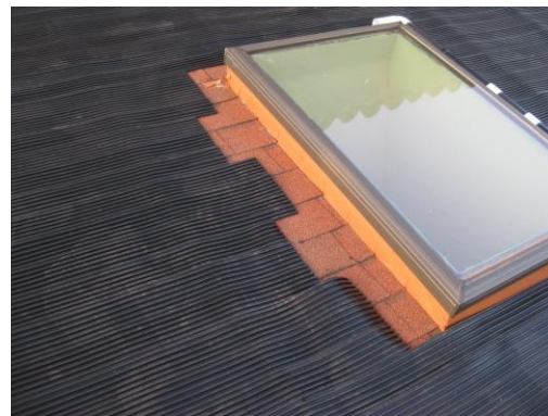
Fin tubing cut before staggered headers attached
