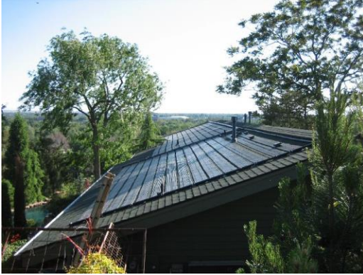
Sideways with alternating headers
