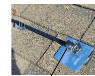
STRAP CLAMP SECURES END
