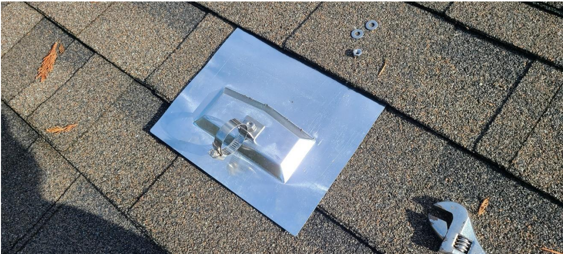
Install the strap bracket, ss washer, 1/4" ss nut and a #20 all ss gear clamp and tighten (the nut).
