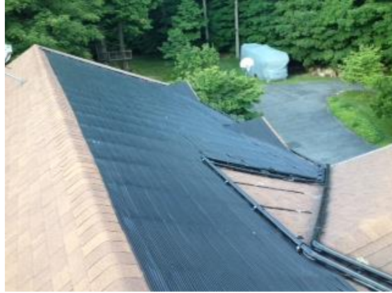
Sideways with staggered headers
