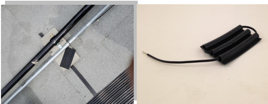
Fig. 2. Hot Sun solar sensor. Don't attach to pipe or solar panel.
