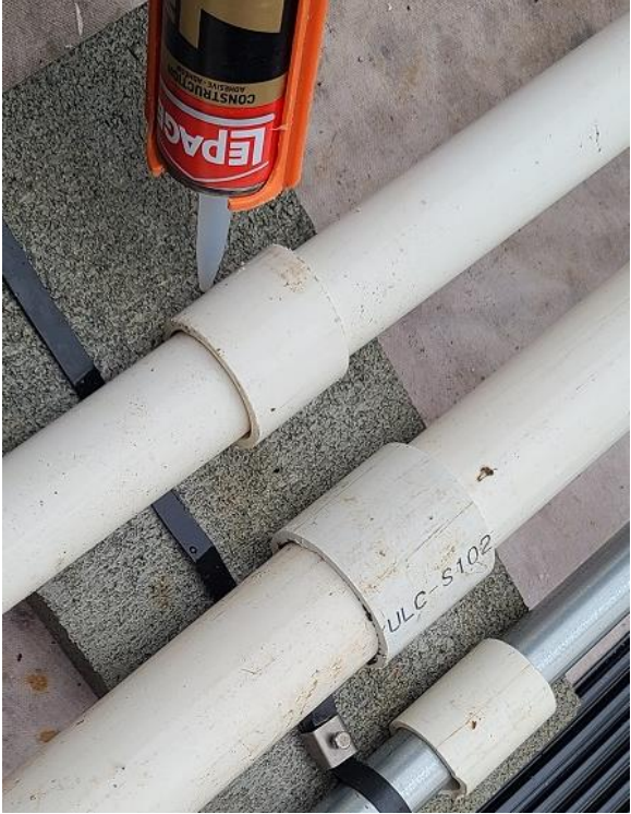
Slip collars glued to ballasts (flat roofs)
