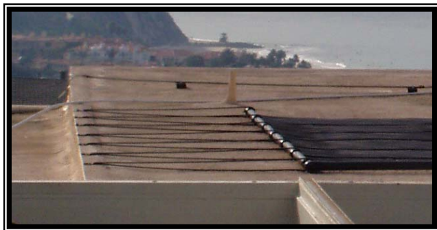
Straps can be lagged onto a parapet wall.
