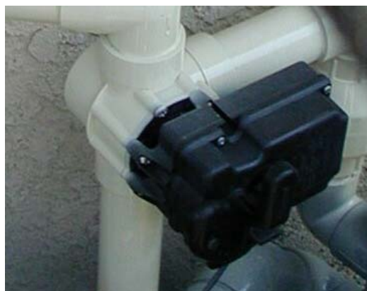
Compool solar valve and actuator.
